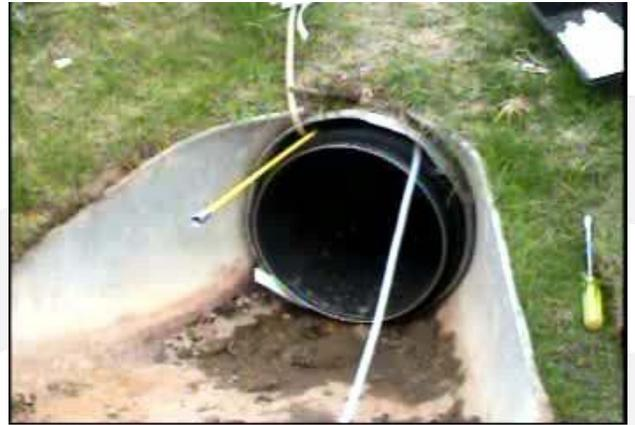
Grout injection into annular space
