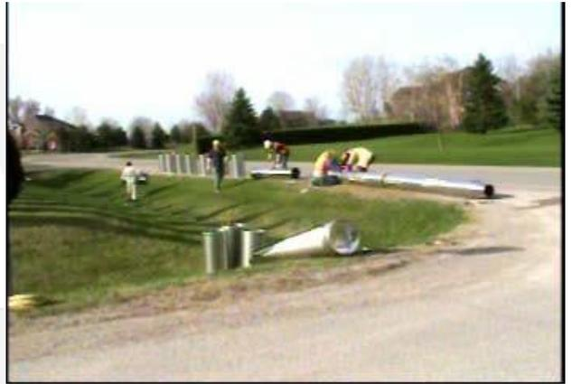
End cone makes it easier to pull the liner into the culvert:
