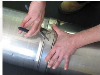
The above sequence of photos of the Insta-Liner<sup>TM</sup> stainless steel core shows two lengths
