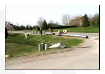
End cone makes it easier to pull the liner into the culvert:
