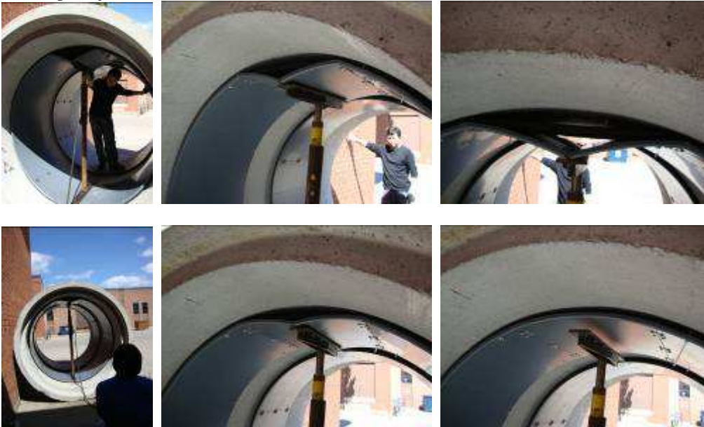
5. Set up the jack for the installation.
