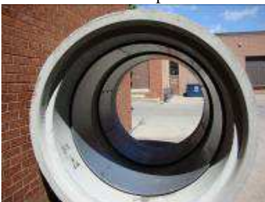
5. Installation is completed.
